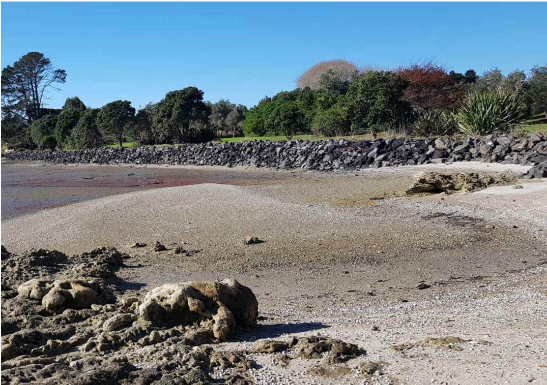
Photo 29 Rock retaining wall at southern end of beach.
